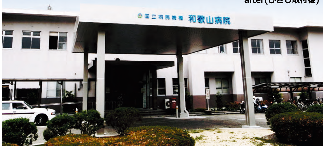
after(ひさし取付後)
